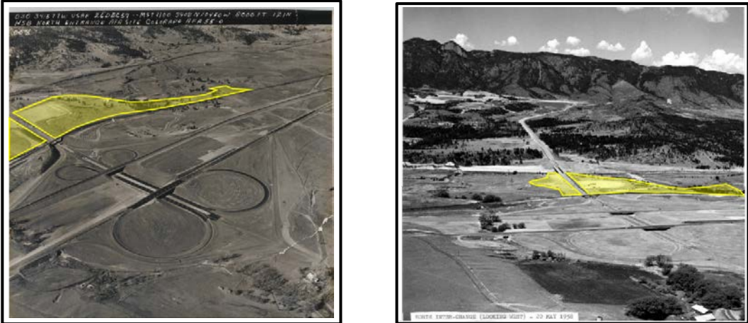
Exhibit 6: (Left) December 1957 aerial photograph of North Gate interchange. (Right) May 1958 Aerial photograph of the interchange. The proposed EUL parcel is highlighted in yellow.
