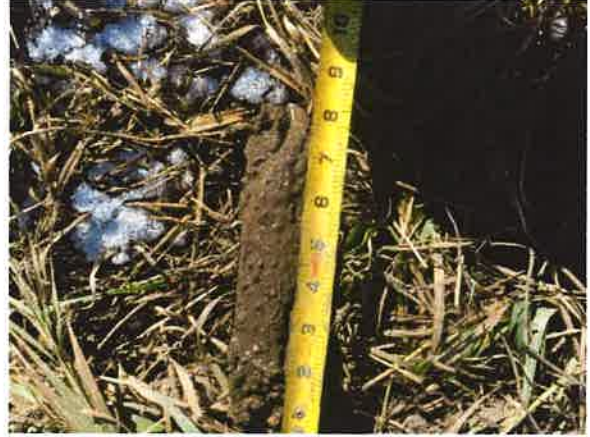
Photo 34 – Community 15 had visible surface water in approximately 80% of the area as well as a hydrogen sulfide odor.
