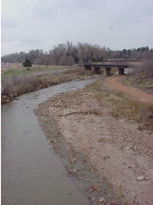
Photograph 24: The Monument Creek (at Bijou Street, Colorado Springs) drainage has a long history of seasonal and at times catastrophic flooding. The drainage has been altered over time to mitigate flooding damage, yet seasonal flooding is part of the creek’s natural cycle.
