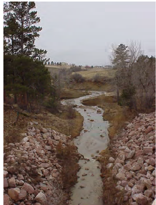
Photograph 8: Most precipitation within the watershed occurs in intense events of short duration, varying widely by season. Increased levels of hard-surface development (streets and driveways) within the watershed, and the presence of highly erosive soils, have resulted in increased levels of sedimentation in regional stream reaches. Smith Creek (above, a tributary of Monument Creek to the east) carries sediment to Monument Creek after an early spring rain shower.
