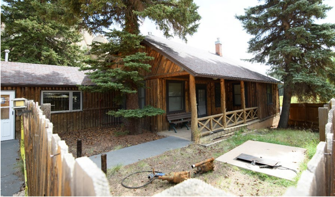
FMRA historic Caretaker's Residence as it appears today.
