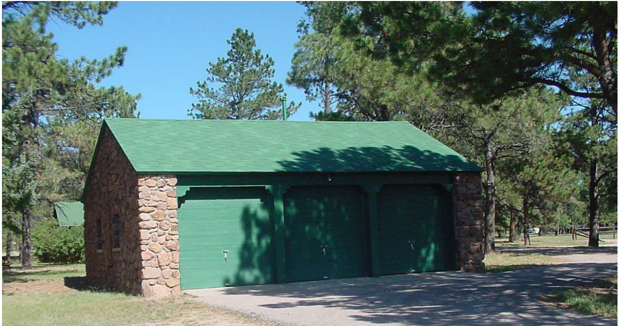
Rose House garage, view West.
