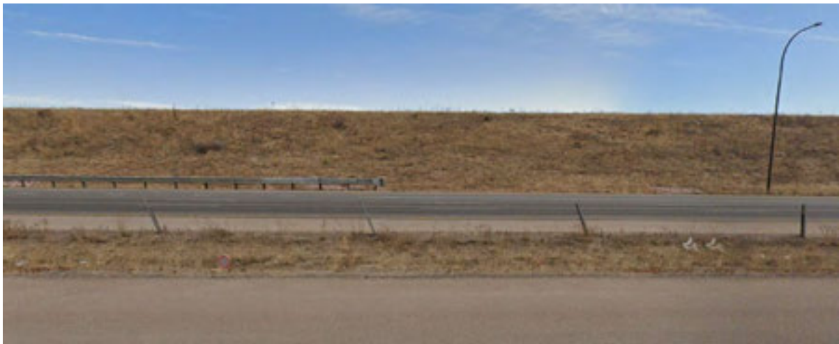
Figure 3: Photograph of Kettle Creek Dry Dam from I-25
