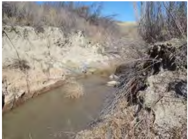
Figure 4: Photograph of Bare Channel Banks with Active Erosion (11/18/2013)
